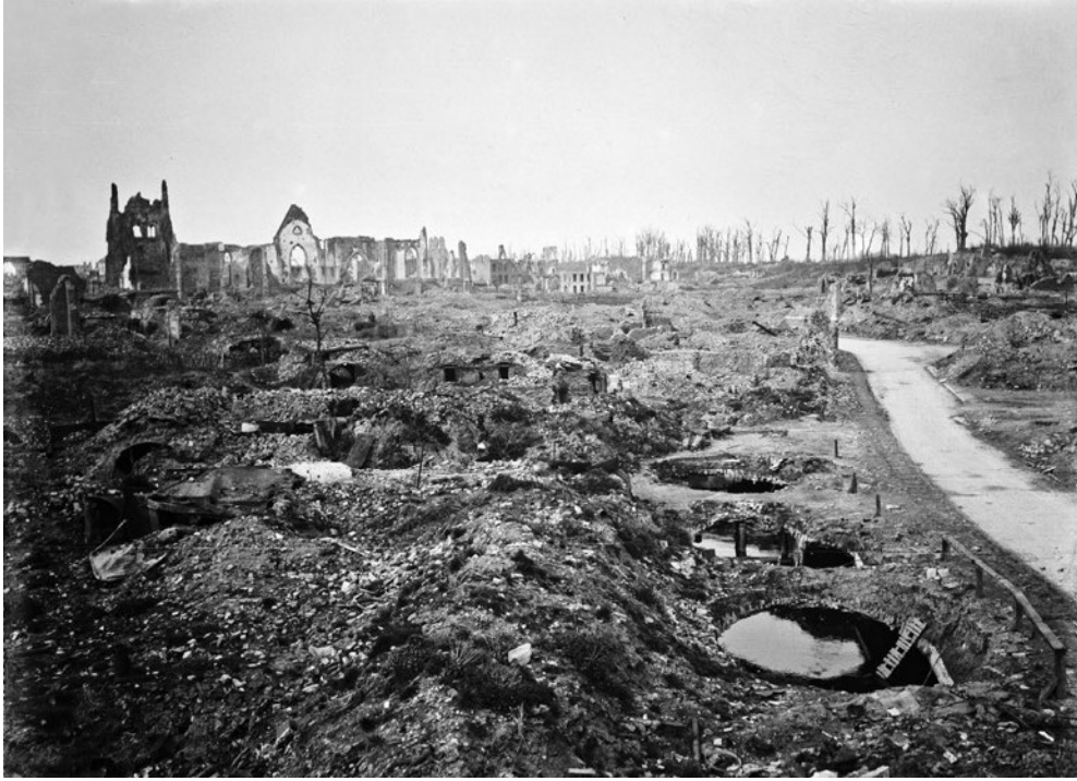
View of the destroyed city of Ypres near the Rijselpoort (Lille Gate), 4 April 1919 (Collection Antony, In Flanders Fields Museum, Ieper).
